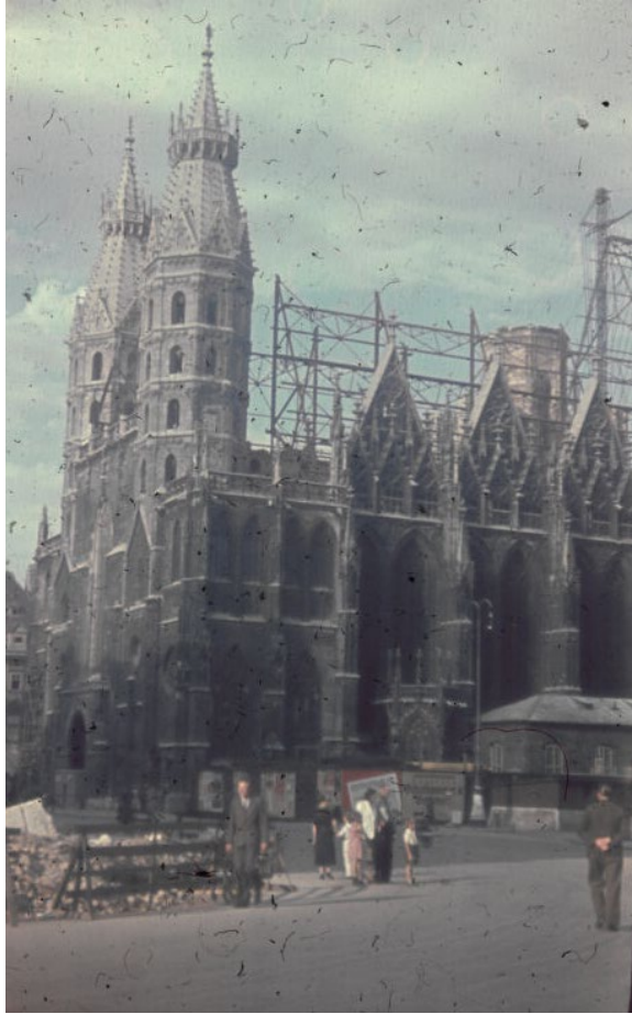
The Cathedral, showing the destruction of the roof after the fire
