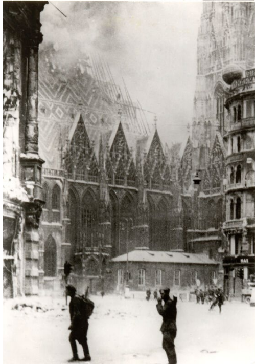
The roof of St. Stephen's Cathedral burns, destroying the Pummerin on 11 April 1945. A 22-ton bomb hit on 12 April 1945, further damaging the South Tower where the Pummerin was housed
